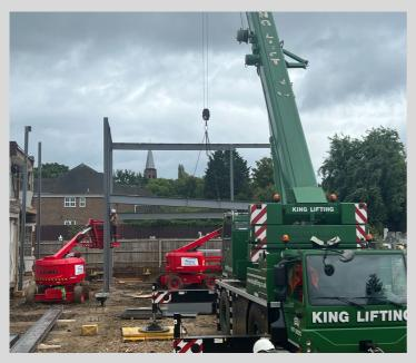
The crane and the red 'cherry-pickers' are the stars of the show along with their deft operators. Each heavy piece is lifted into place by the crane followed by a pincer movement as the two cherry-pickers move in and up on either side, to secure it to the adjoining steel.
